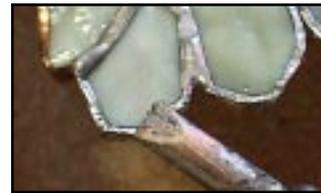
Next, flux an area you can comfortably finish soldering before the flux can evaporate. Start at the top of the piece and work down. This prevents you from dragging your sleeves and hands through the flux.
