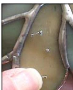
You may find small pieces of solder stuck to the glass. You can easily remove these using your fingernail, or 000 steel wool. Be careful not to scratch the glass.
